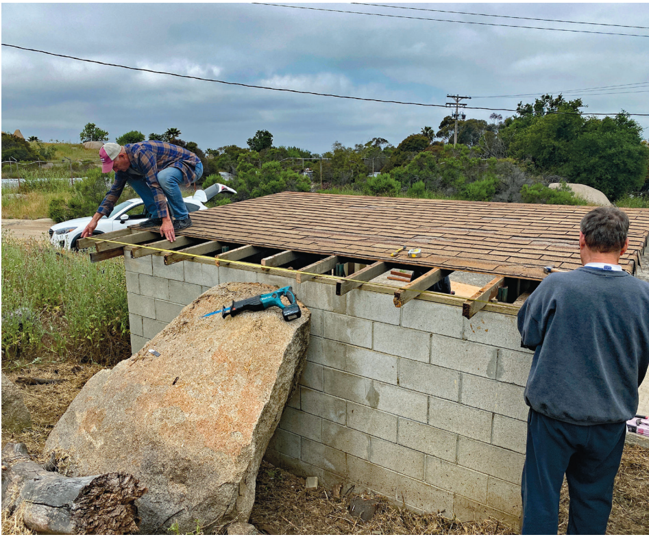
David Roberts and Tom Green repairing the roof on the shed
